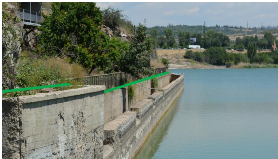
Figure 7: Position of cable on the spillway up to the dam substation
