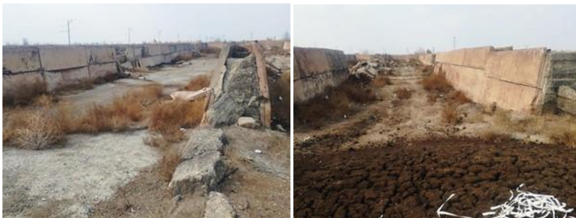
Figure 13 – Former WWTP (left) and solid poultry manure storage (right)
