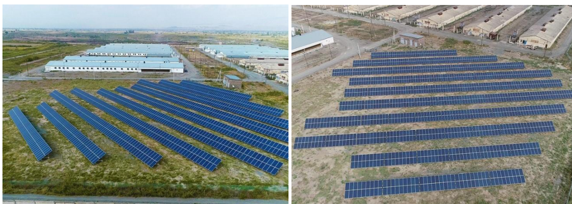
Figure 11 – On-site solar power plant 500kW
