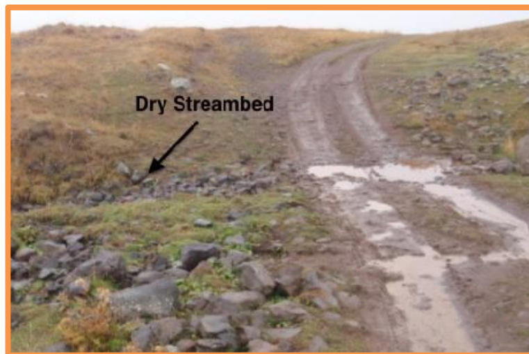
Figure 1-4. Dry Streambed across Existing Road 10km from M2
