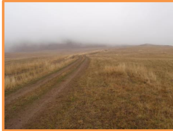
Figure 1-3. Existing Rural Road 4km from M2
